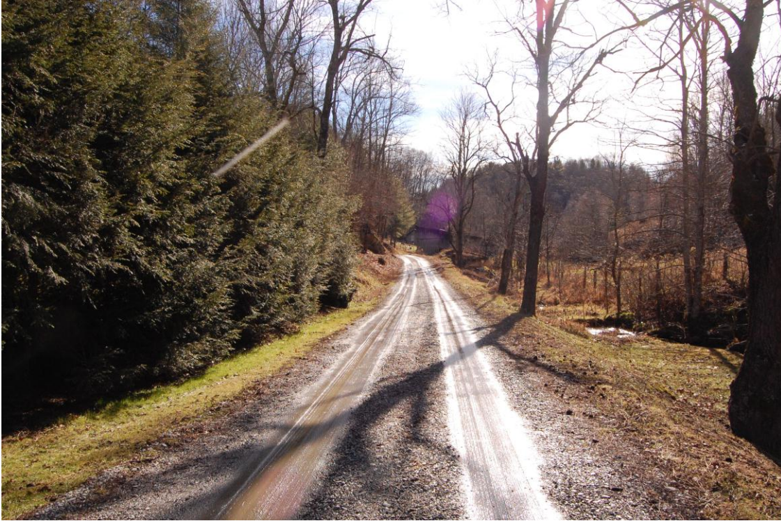
Figure 4: View to the south-southeast from Bridge No. 428 along Jim Duvall Road
