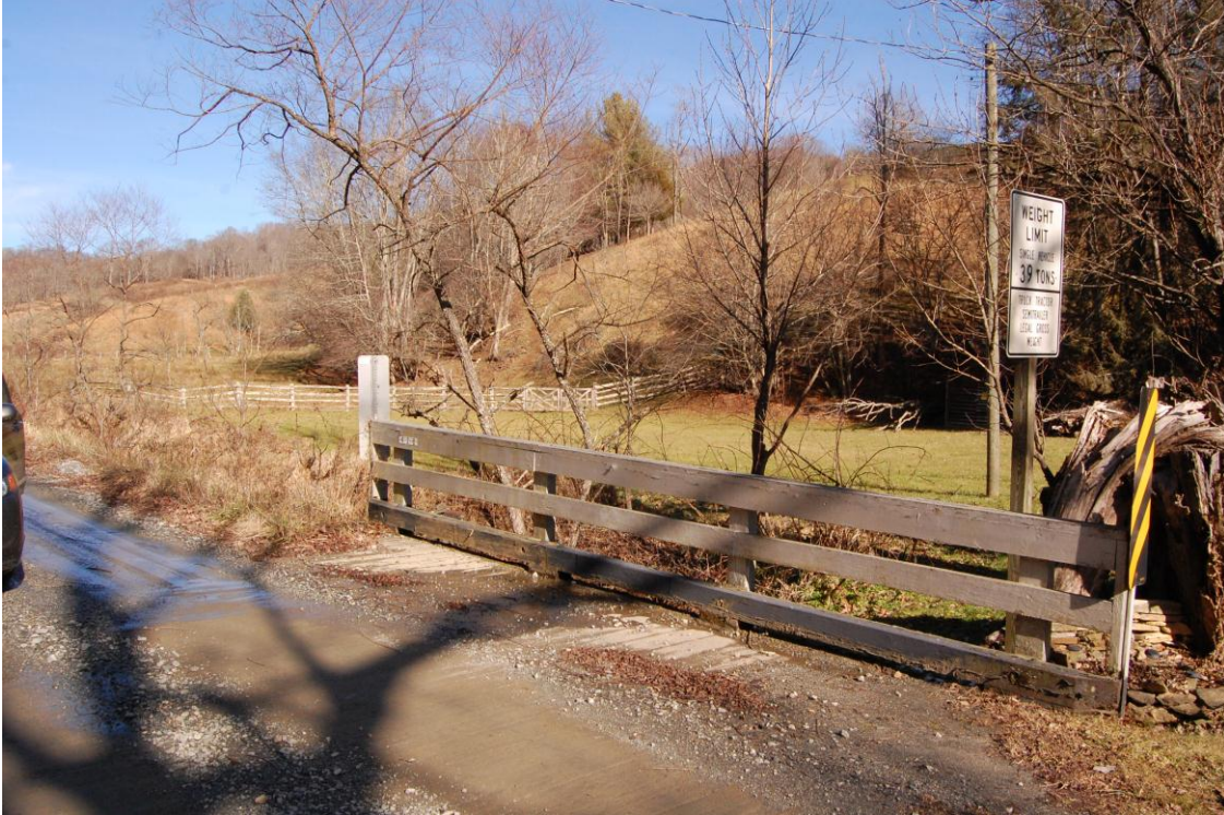
Figure 2: Bridge No. 428 over Long Branch, view to the northeast
