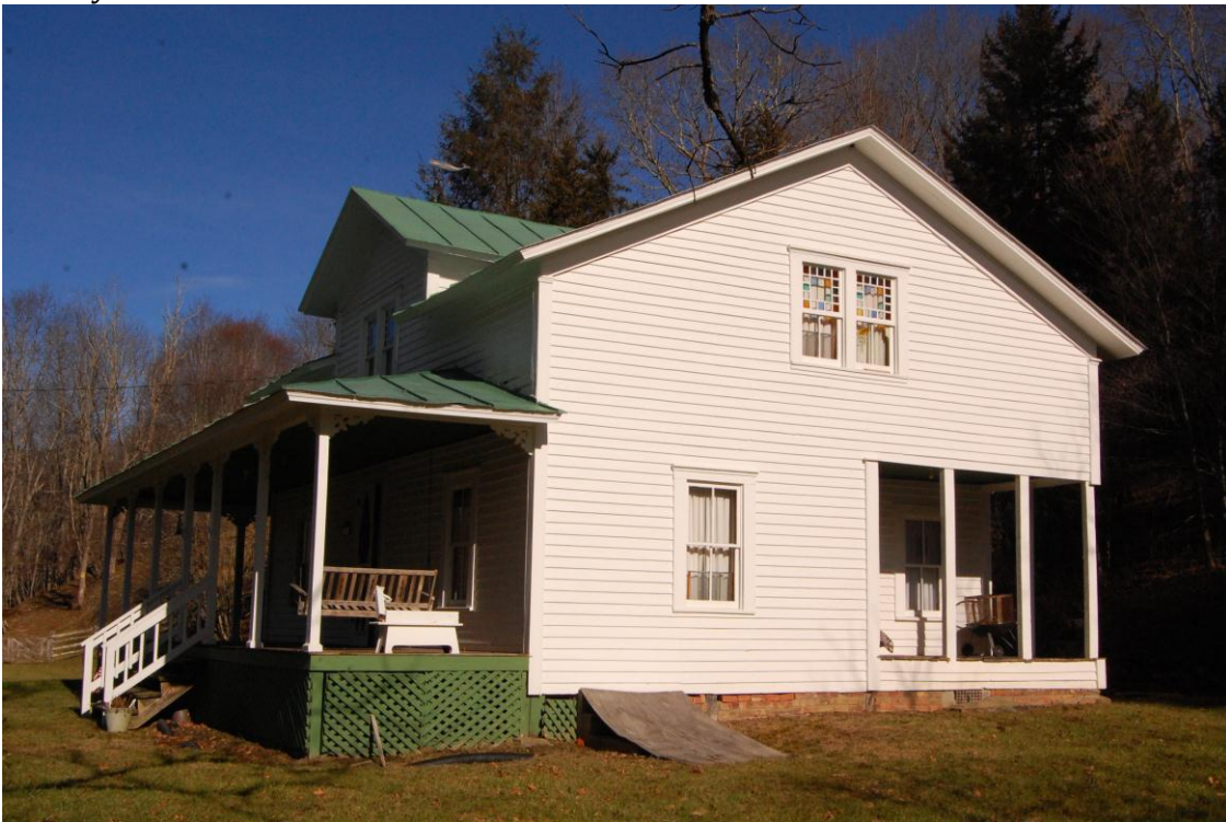
Figure 6: Jim Duvall House, south elevation, view to north-northeast
