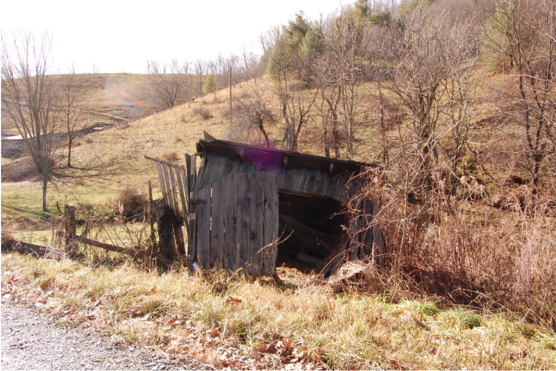
Figure 13: Shed facade, view to the southwest
