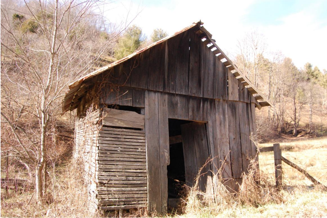
Figure 12: Crib facade, view to the west-northwest
