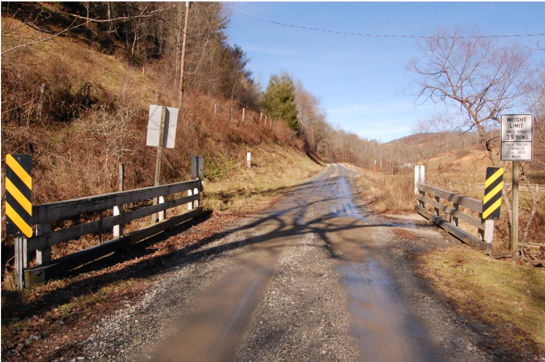
Figure 3: View to the north along Jim Duvall Road and Bridge No. 428
